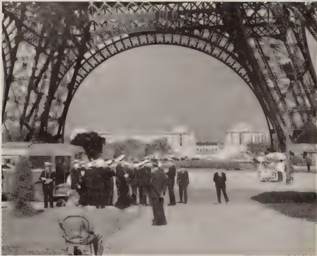
The base of the tower
